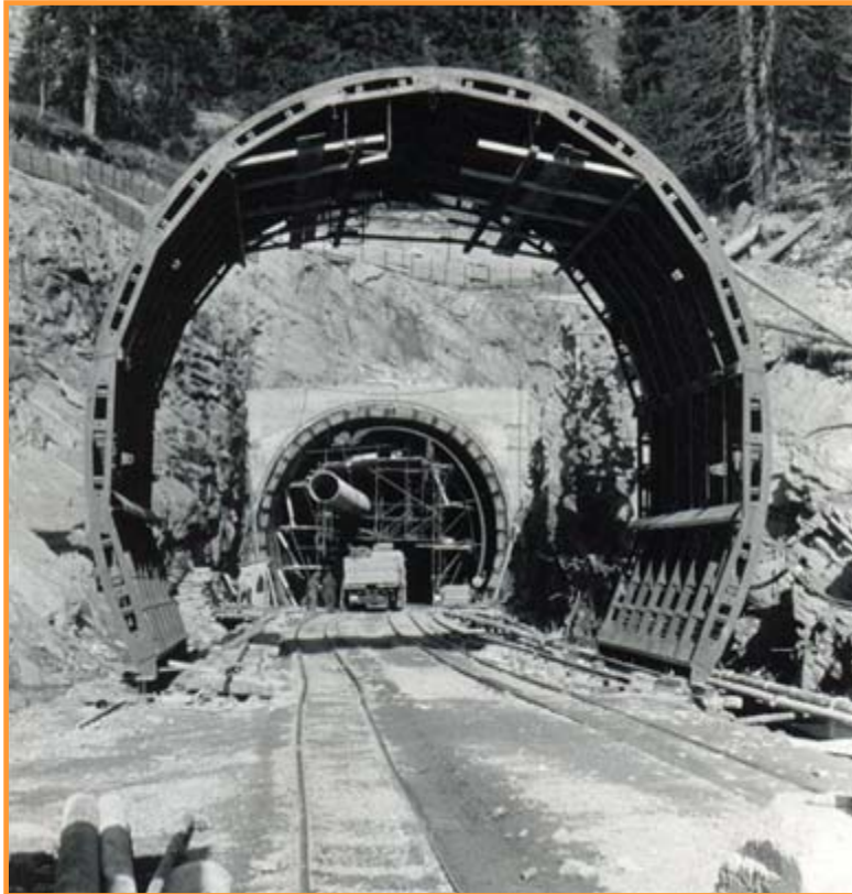
Tunnel San Bernardino (1962/66)
