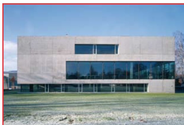
New building single-family home, Hergiswil, NW-031
